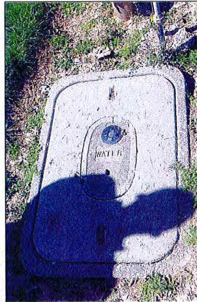
Figure 3 Sensus 520M FlexNet SmartPoint Radio Transceiver and Typical Installation
