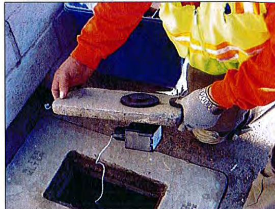
Figure 3 Sensus 520M FlexNet SmartPoint Radio Transceiver and Typical Installation
