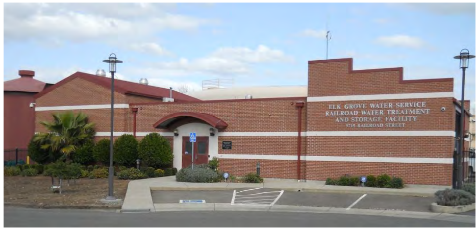
The Railroad Water Treatment and Storage Facility
